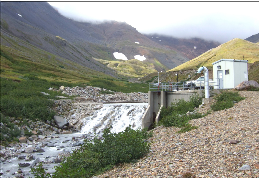
King Cove's Hydroelectric facility at Delta Creek
